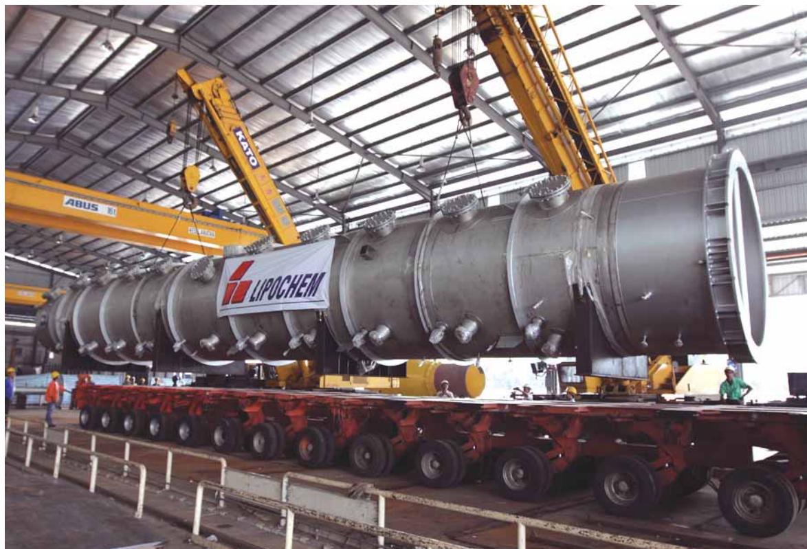
Engineers at Lipochem are busy preparing a distillation column to be shipped over to Indonesia and installed there. New refineries are a lot bigger and are erected at a faster pace.
